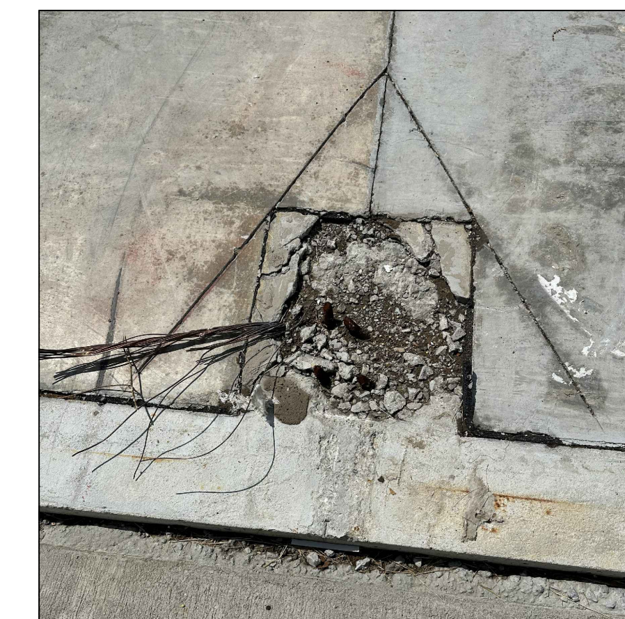
MAIN COLUMN PEDESTAL DAMAGE
